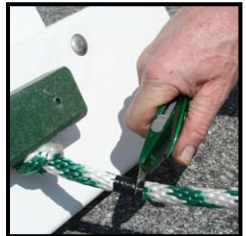
If the rope is too long, wrap tightly with black tape. Then with a utility knife, cut into the tape to separate the excess rope.
